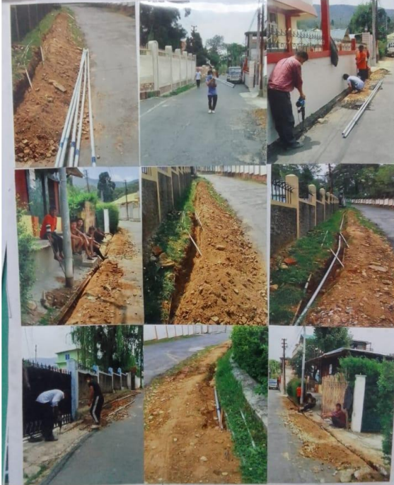
NEW DISTRIBUTION SYSTEM DURING CONSTRUCTION
